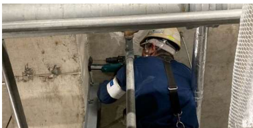
Fig. 7 Drilling holes in the concrete structure
