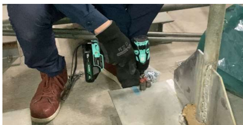
Fig. 6 Tightening of nuts
